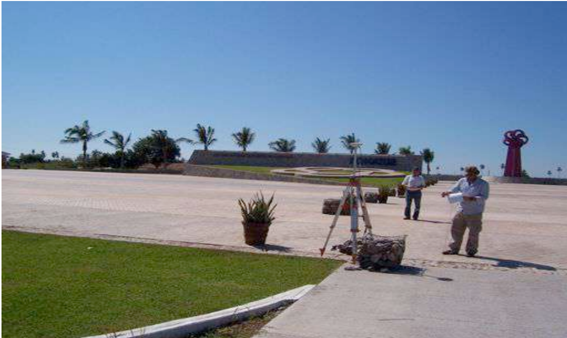
ABGPS located at the project site – ESC1
